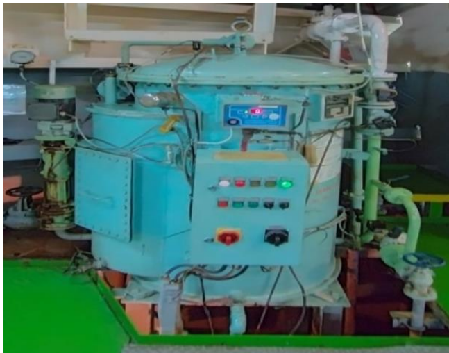
Gambar 2.1 Oily Water Separator (OWS).
