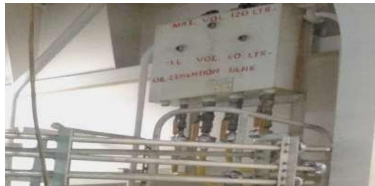
Gambar 2.12 pipa-pipa *oil reservoir tank*
